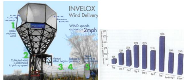
(a) The invelox wind energy system (b) p.u. captured energy for a given site
